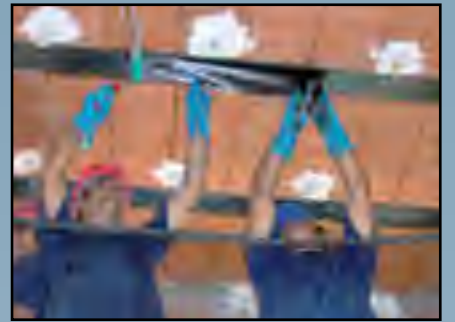
JOISTS AND PRECAST BEAMS. Mercadona. Plaza de la Remonta (6.500 m 2 )
