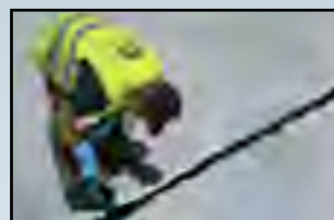
CONCRETE SLABS JOINTS Base Militar de Albacete, (10.000 m)
