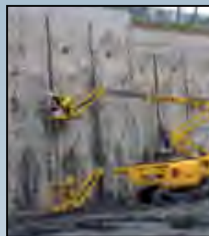
RETAINING WALLS JOINTS ACCIONA Sede Pegaso Madrid, (2500 m)
