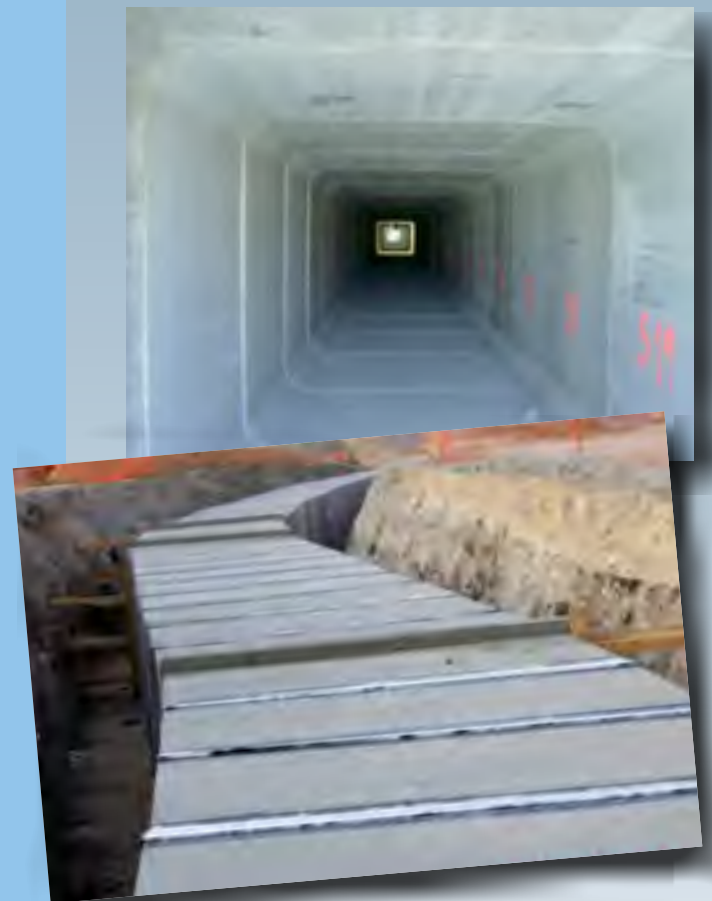
Sacyr Collector M-45 ring highway Joint sealing (100.000m)
